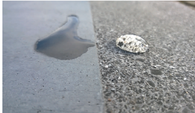
Left: untreated fair-faced concrete
