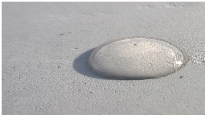
Fair-faced concrete protected with COLORTEC® finish
